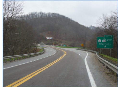
Mountain Parkway Extension Exit 75
